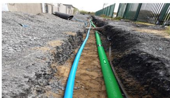
Installation of water mains & Telemetry duct
